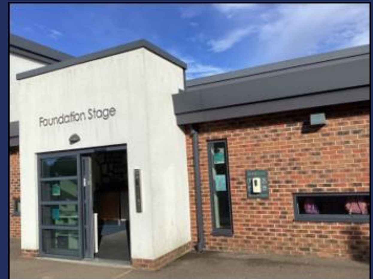
The Foundation Stage Entrance
