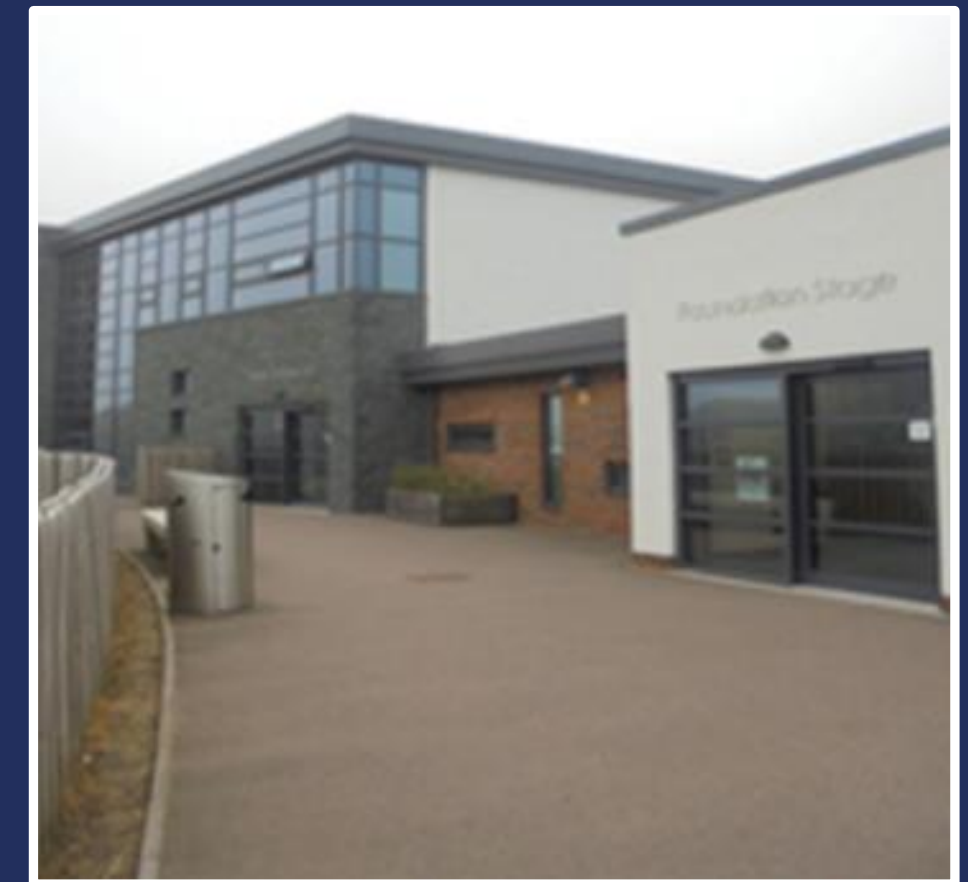
The Foundation Stage Entrance
